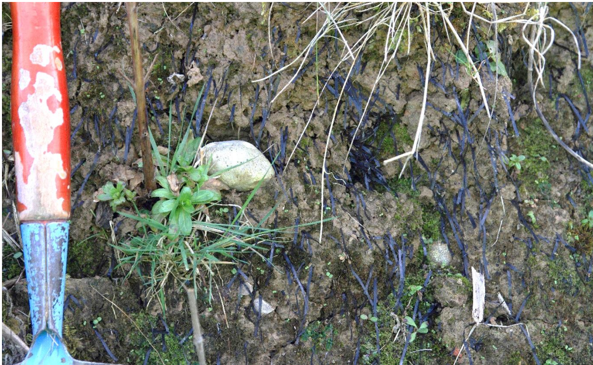
Figure 5: Fibres entrained within the soil of the back scarp at A27 Polegate/Bay Tree Lane FRS trial (Site Photograph 7DW_4191)
